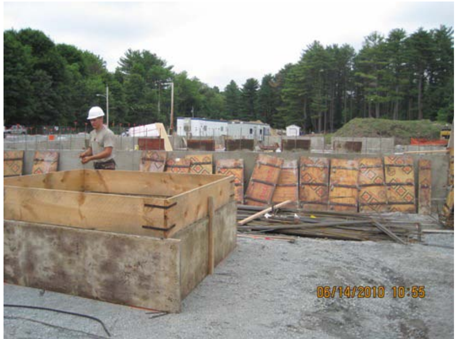
Formwork for interior footing
