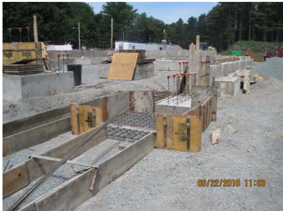
Formwork and reinforcing for spread footings 12 line
