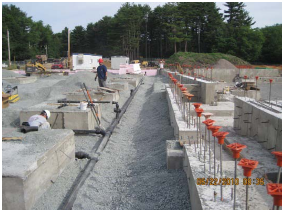
Completed foundations and layout of underground plumbing along 7 line
