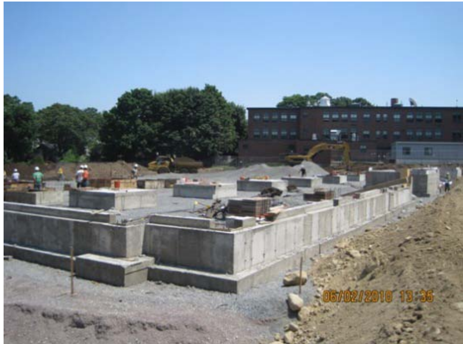
Completed foundation wall along 1 line
