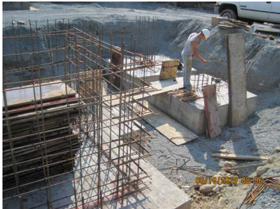
Interior footings and foundation wall steel reinforcing
