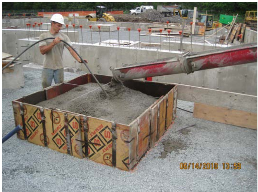
Pouring interior footing
