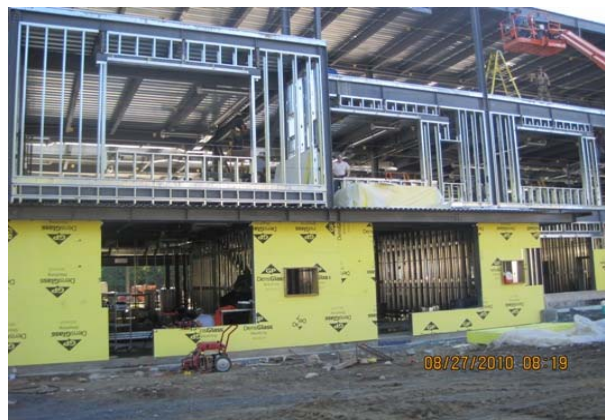
Exterior framing and sheathing
