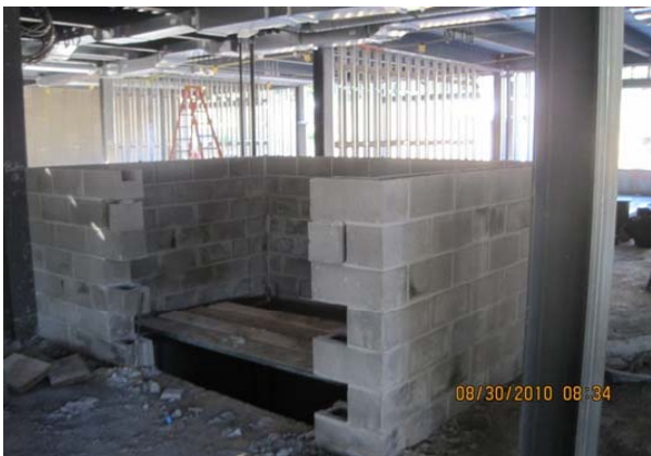
Elevator Pit CMU
