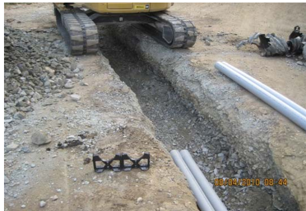
Main electric duct bank trench
