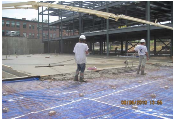
Slab on Grade placement
