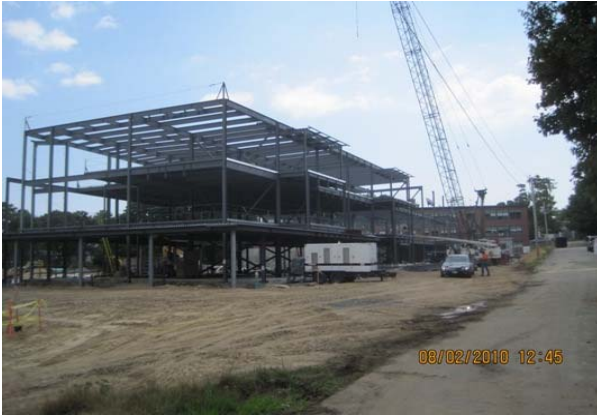
Erection complete west side of building
