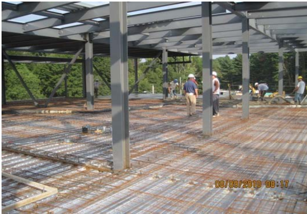
First floor Slab on Deck
